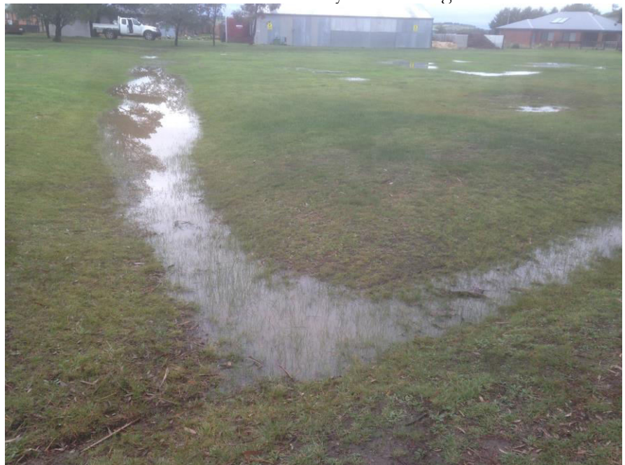
Drain on 6 th fairway not clearing.
